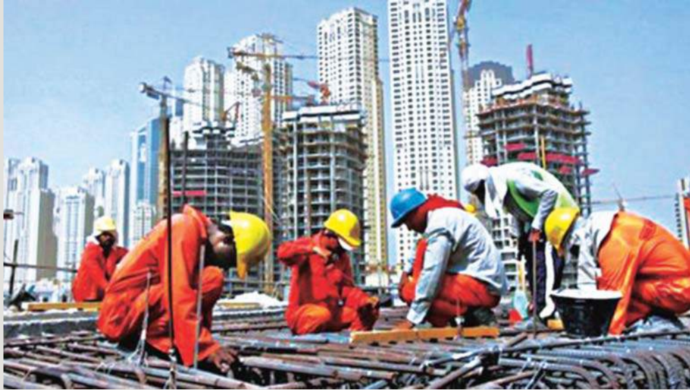
Bangladeshi labour force working at construction site in Dubai
