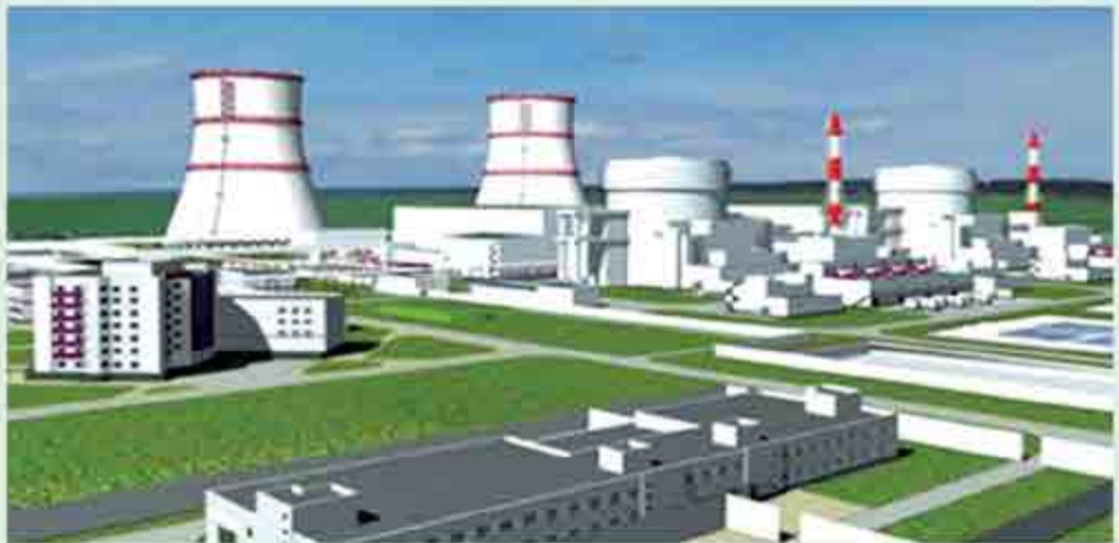
Rooppur Nuclear Power Plant under construction at Pabna
