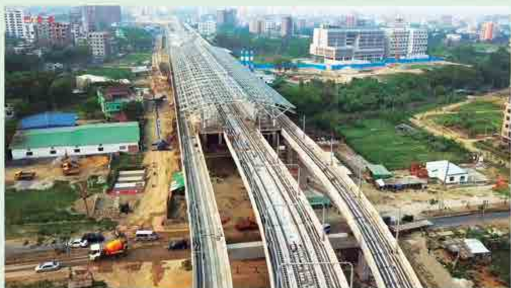
Metro Rail Project under construction in Dhaka
