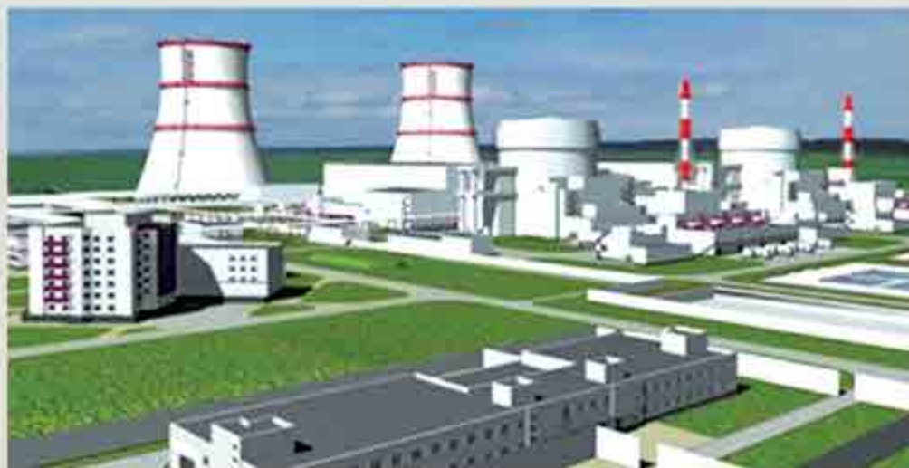
Ruppur Nuclear Power Plant under construction in Pabna
