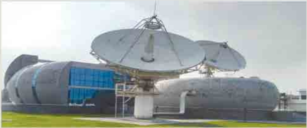
Bangabandhu-1 satellite ground station at Gazipur
