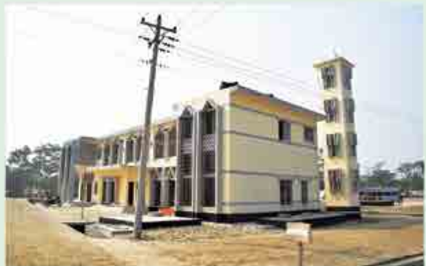
Mosque and Eidgah in the rehabilitation complex
