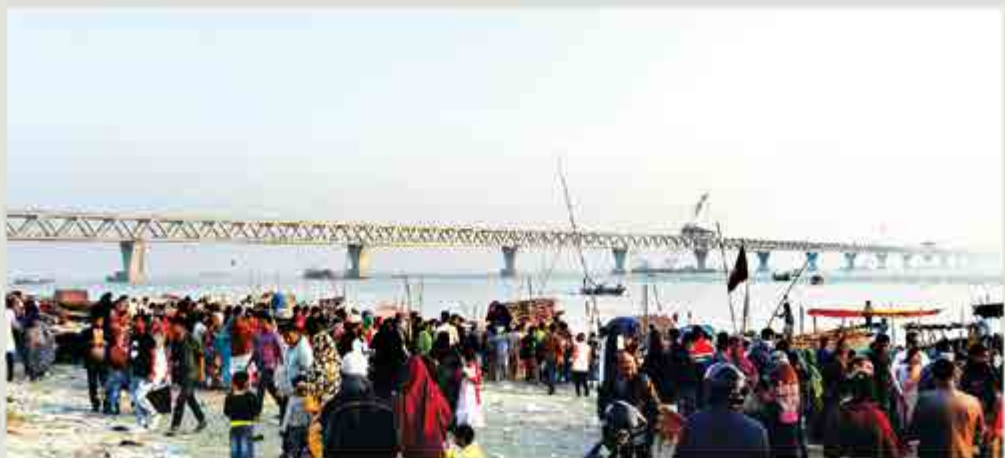
Padma bridge, the largest river bridge of the country, is being constructed by gov't own funding.
