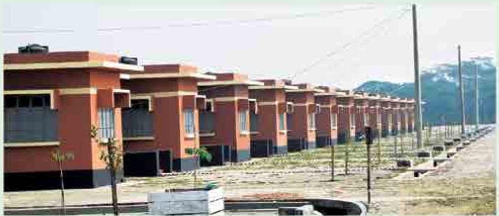
Houses built for the affected families of Payra port.
