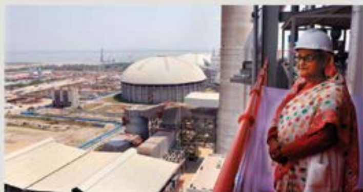
Prime Minister Sheikh Hasina inaugurates the country's largest 1320 MW Payra Thermal Power Plant at Patuakhali on March 21
