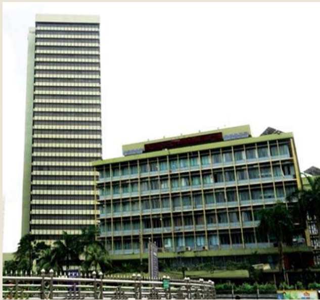
Bangladesh Bank (Central Bank of Bangladesh), Dhaka
