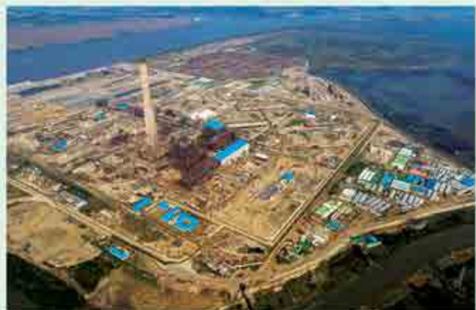
Rampal Coal Power Project
