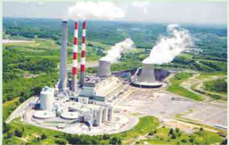
Matarbari Power Plant
