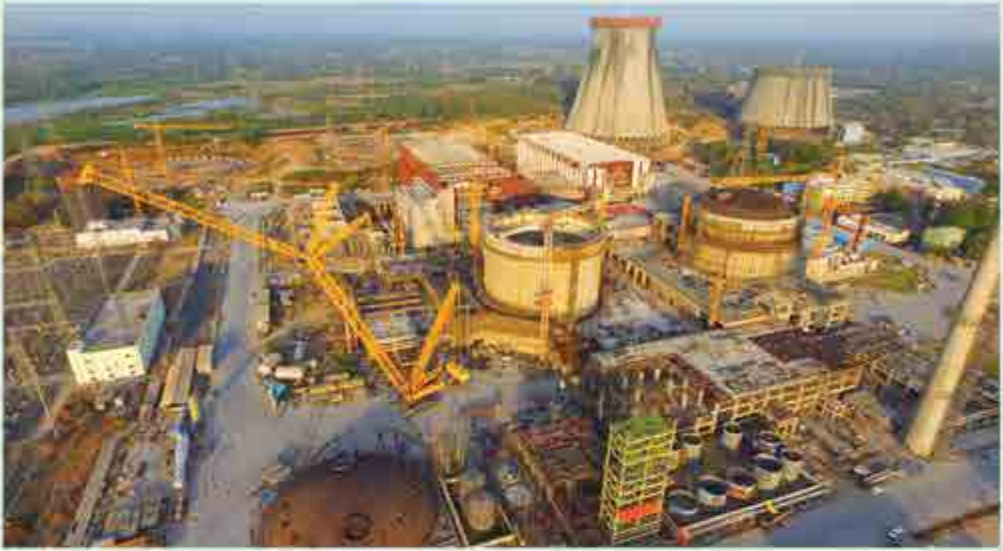
Rooppur Nuclear Power Plant
