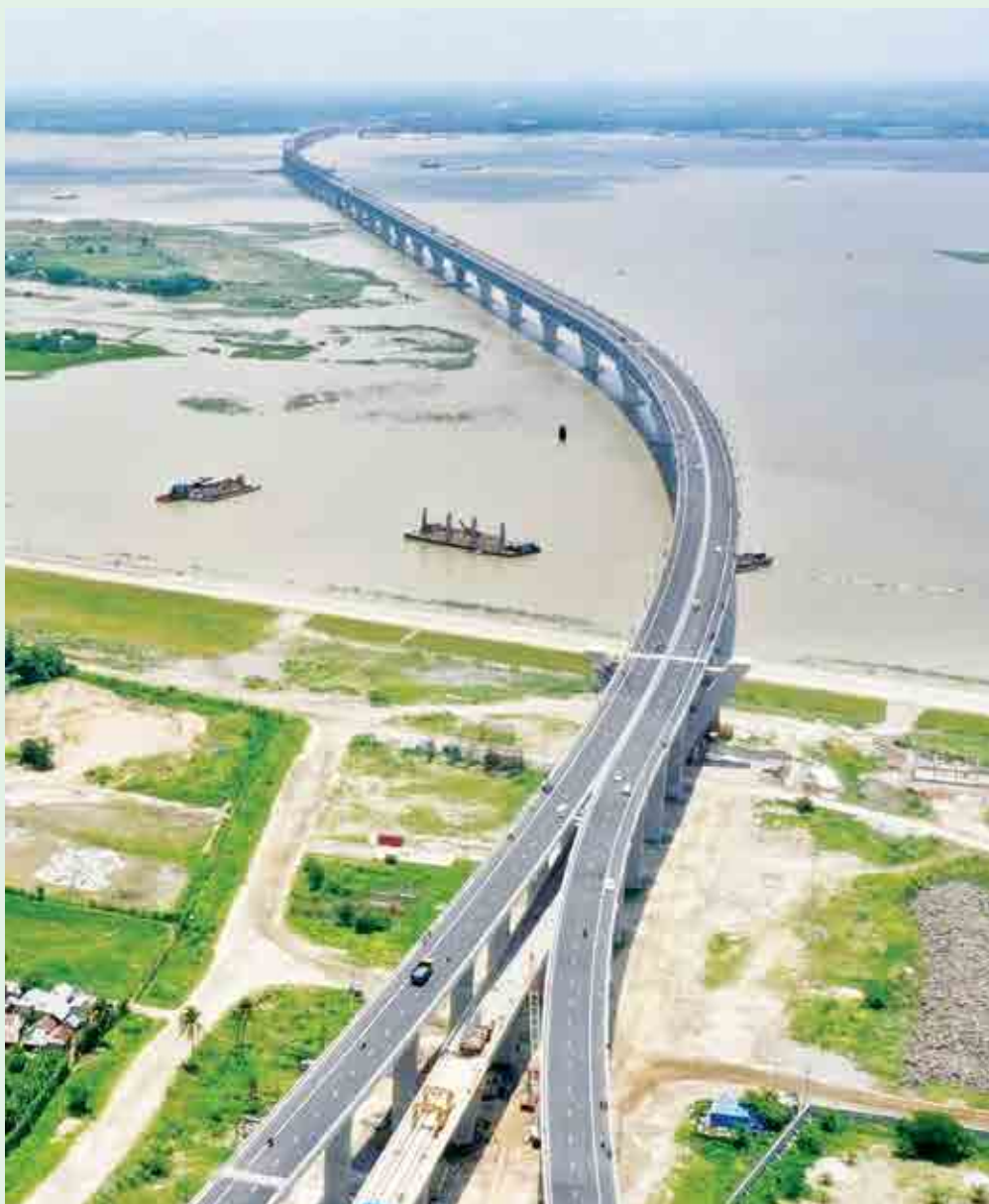
The Padma Bridge at the Mawa point in Munshiganj district
